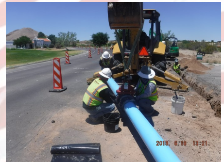
Crews from Morrow Enterprise installing new water lines along Via Norte
