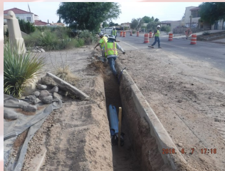
Crews from Morrow Enterprise installing new water lines along Via Norte
